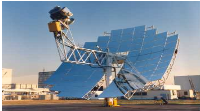
Figure (3.3): A parabolic solar collector concentrating the sun's rays on
